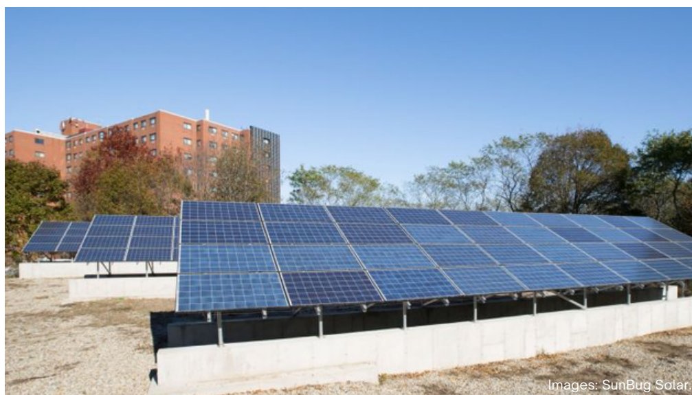
Proposed 23.9 kW rooftop array (top left) and 63.5 kW rooftop array (bottom left). Existing 120-panel 27.6 kW ground array located on site (right). Images: SunBug Solar.
