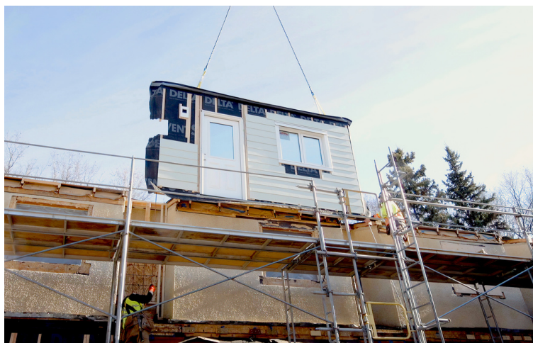
Sundance Housing Co-op townhouse during renovations.
