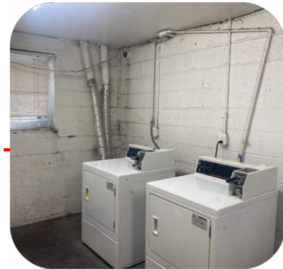
Existing vented gas dryers
